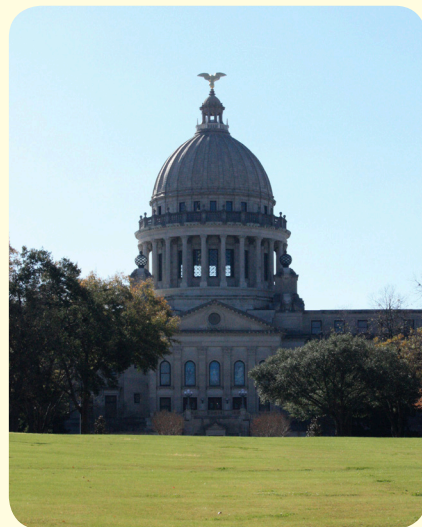
The Mississippi State Capitol Building, photographed on November 30, 2012.
